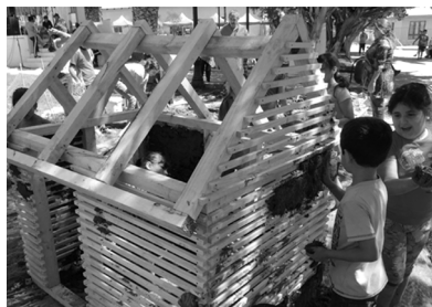
Figure 6 – Creating a half-sized house using reclaimed adobe in a quinchá construction technique
